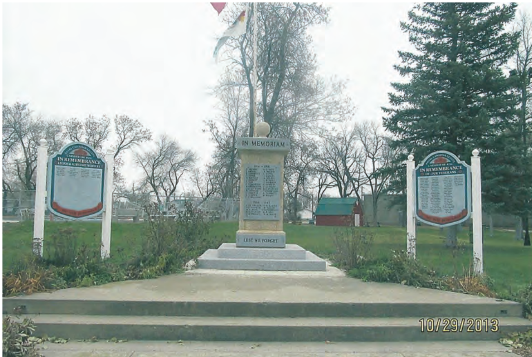
Cenotaph after renovations
